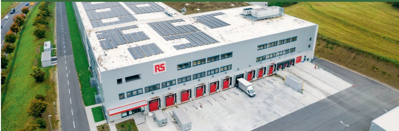
Our upgraded distribution centre (DC) in Bad Hersfeld, Germany, is powered in part by a 6,000m 2 solar array which generates 750kW of green photovoltaic (PV) electricity and 22% of the site's annual electricity requirement. The expanded site can now house up to 500,000 products, which will significantly reduce delivery distances and associated transport emissions.
